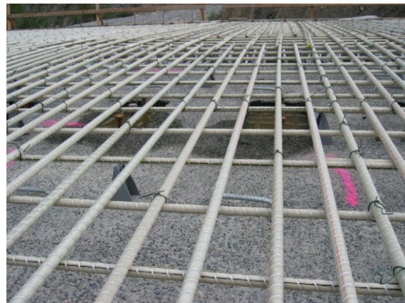
Figure 5.15 – FRP reinforcement in a road bridge deck (Hughes Brothers).
