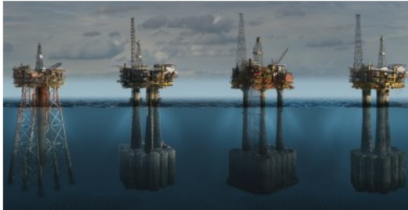
Figure 5.13 – Prestressed concrete offshore platform substructures ( www.constructionenquirer.com/2015/02/03/shell-plans-to-dismantle-brent-oil-platforms/ )
