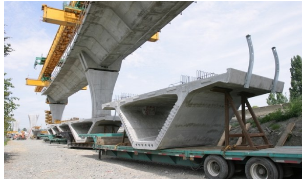
Figure 5.12. Segmental, precast, post-tensioned bridge construction ( www.bethlehemconstruction.com/sw/concrete/segbridge/ )
