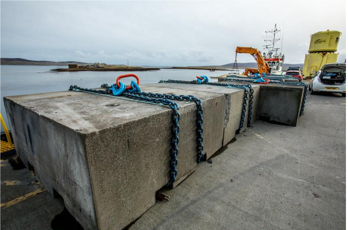
Figure 9: Dense concrete blocks to ballast anchor frame. Each block weighs 22t
