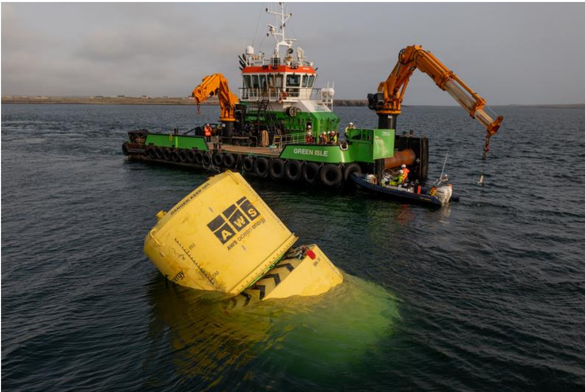
Figure 2: Waveswing during installation in Scapa Flow
