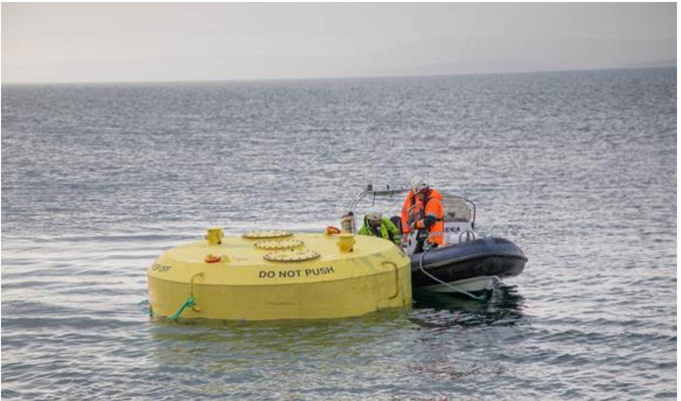
Figure 12: Waveswing during submergence operation
