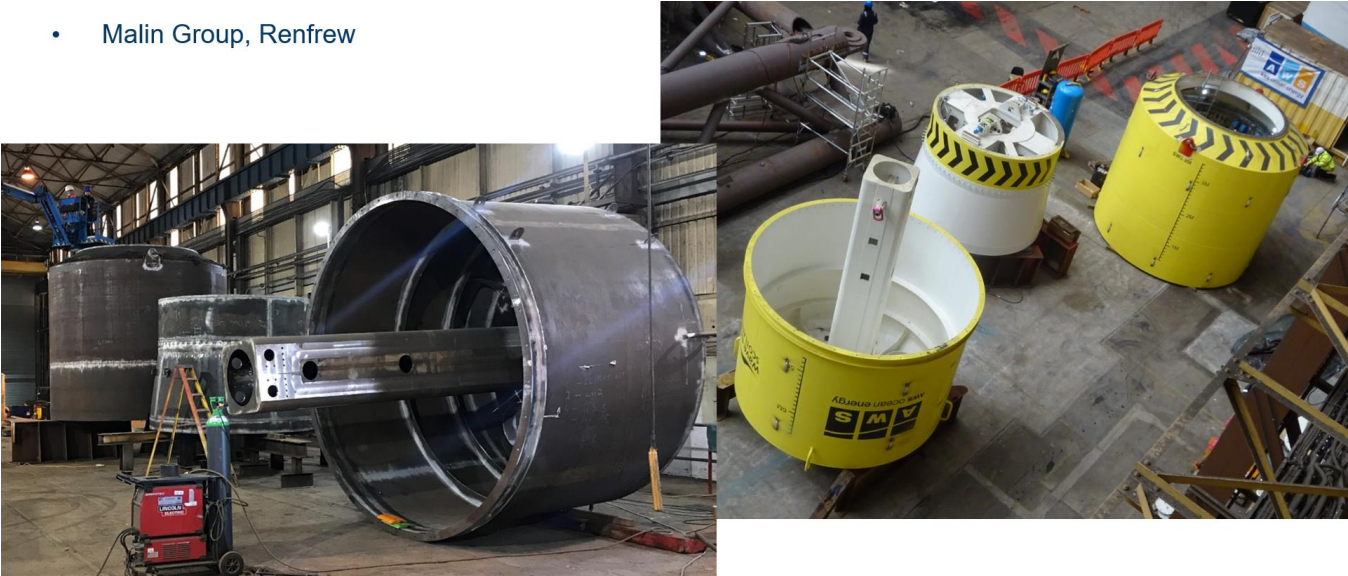
Figure 5: Major fabricated components in Malin's factory in Renfrew
