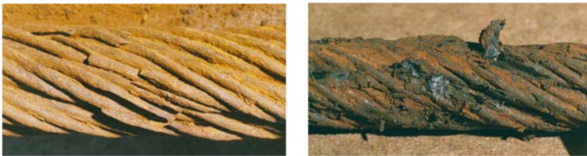
Figure 12: (left) Corrosion and break-up of independent wire rope core (IWRC) of 76 mm ungalvanised MODU mooring rope after five years' service; (right) IWRC of 90 mm galvanised MODU mooring rope after 7 years [31].
