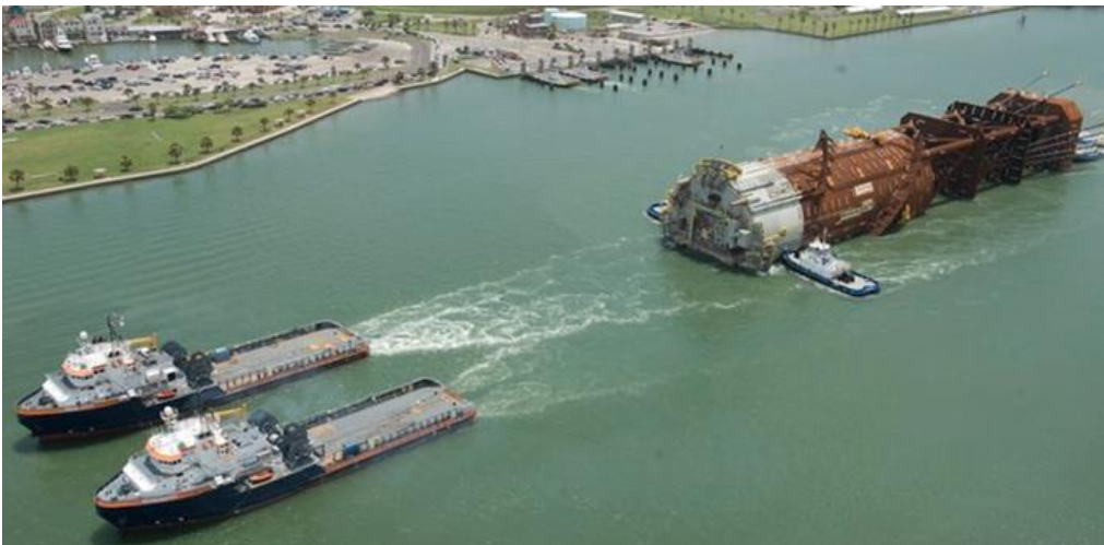
Figure 55. Multiple tug tow-out of a ~180m truss-spar using multiple tugs
