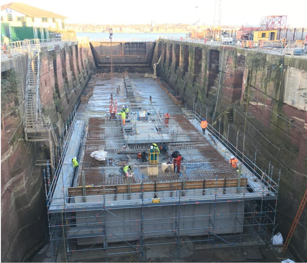
Figure 20. 1250te concrete caisson under construction in Cammell Laird Dock 4
