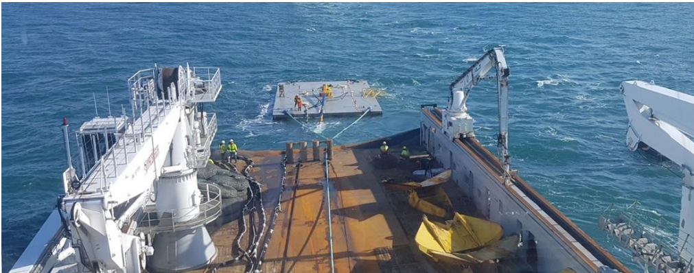
Figure 54. Single tug float-out of a concrete gravity substructure (L21.5m x W2.75m x H4.65m)
