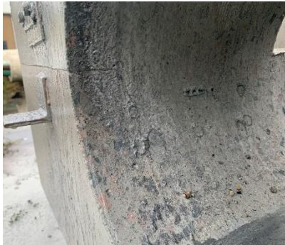
Close up view of extracted core across the precast connection
