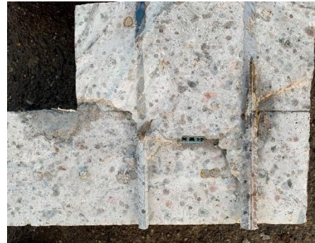
Split core showing no water penetration past the midpoint of the section
