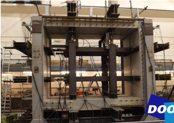
Precast Concrete Connection: Watertightness Testing
