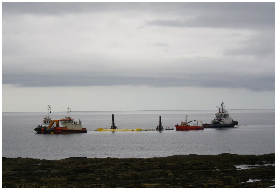
Figure 5 – Installation of Oyster 800
