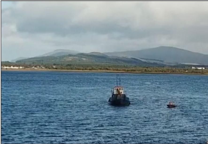
Figure 1 - Installation equipment (showing Loch Shiel and Ben Chrom vessels)
