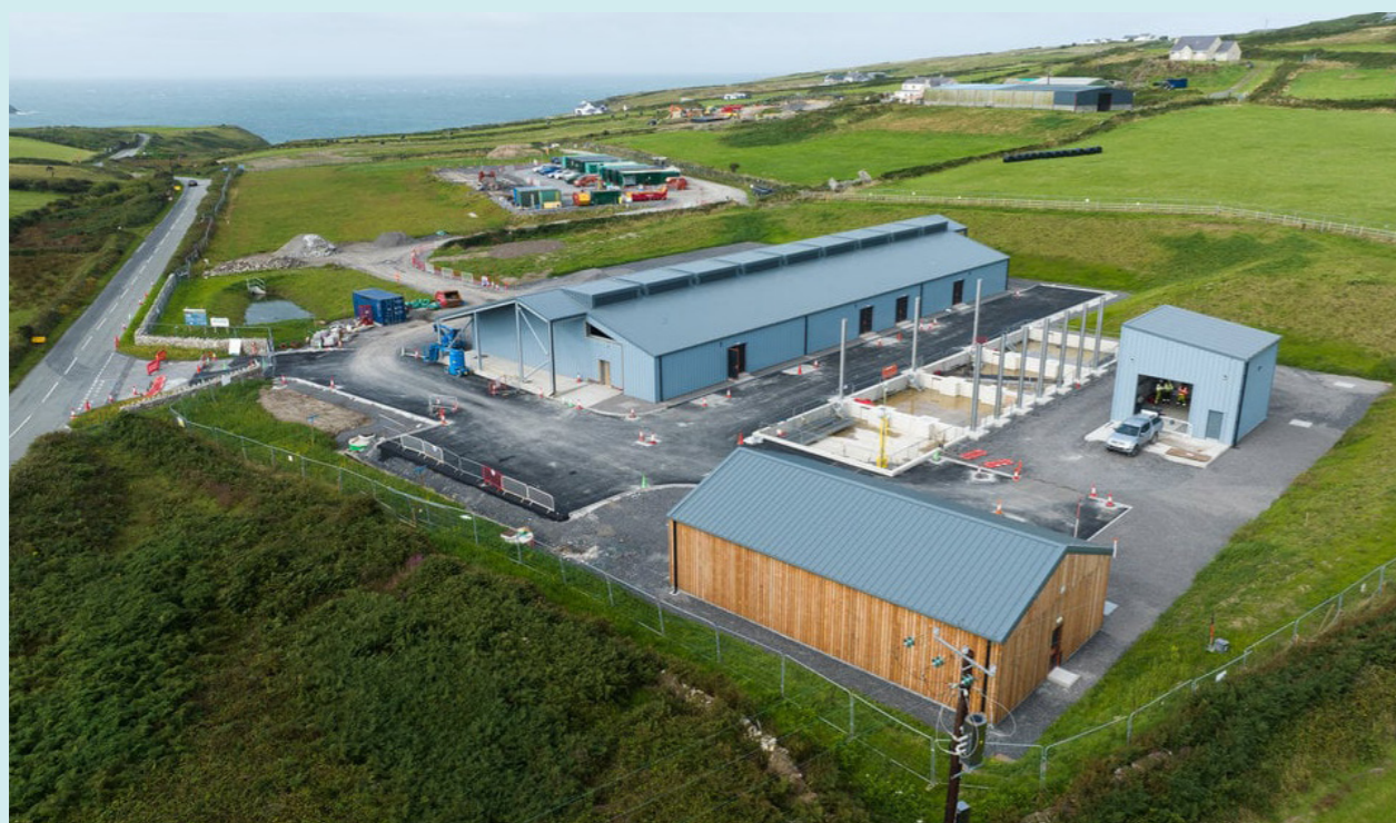
Morlais onshore substation under construction (Credit: Morlais)
