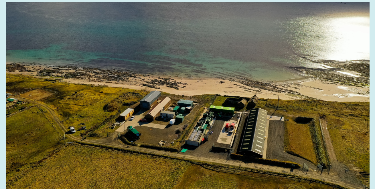
EMEC Caldale substation and storage site looking out to Fall of Warness (Credit: EMEC)
