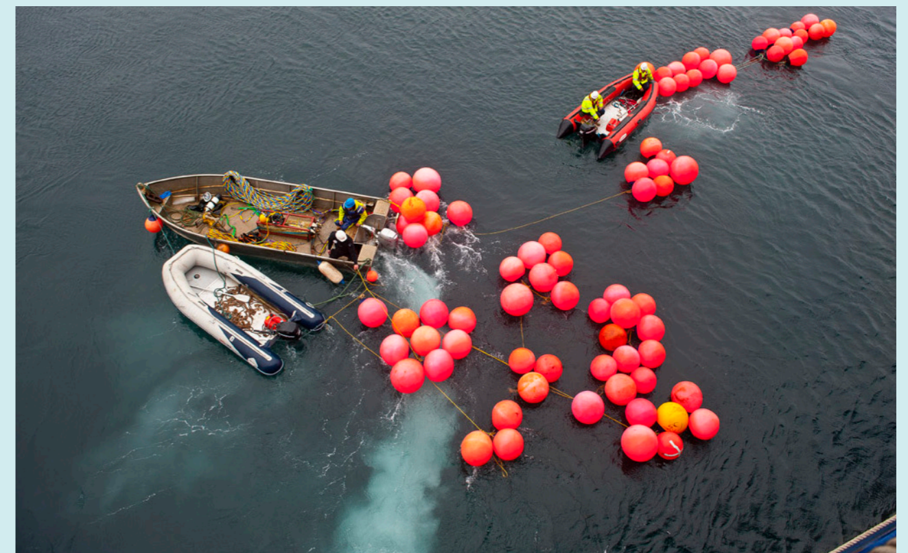
EMEC cable laying operations (Credit: EMEC/ Mike Brookes Roper)
