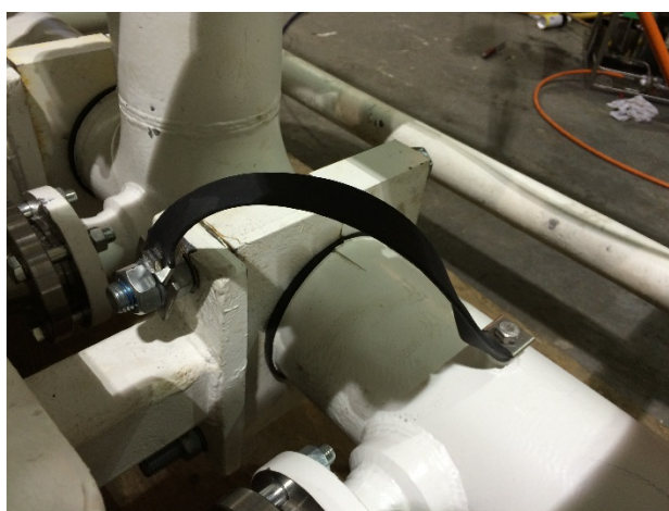
Figure 8 – Example of good continuity cable design. Short span, flexible wire weave, plastic protection around weave, crimped ends bolted to parent components.
